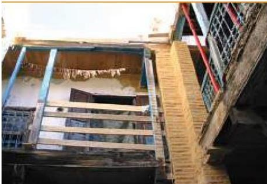
Figure 3: rebuild of a traditional masonry pillar
