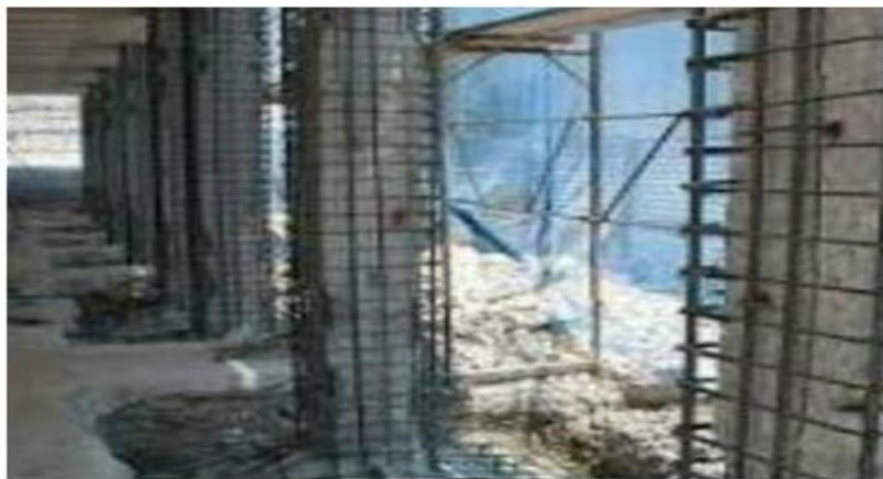
Figure 16: Lining of reinforced concrete columns
