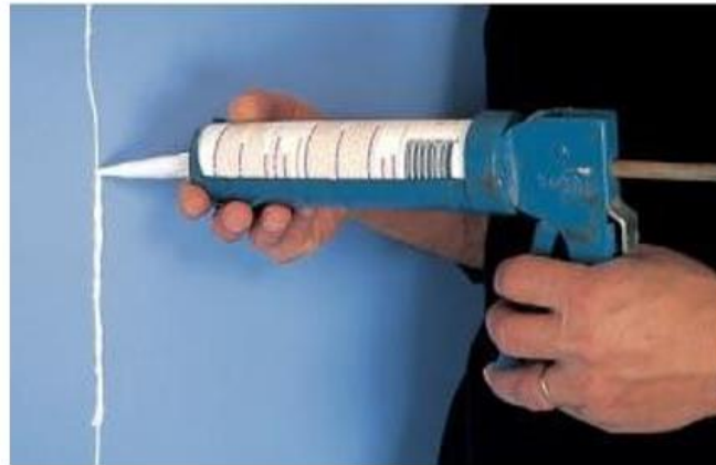
Figure 23: Repair of Cracks in Wall with Epoxy-Based Coating.
