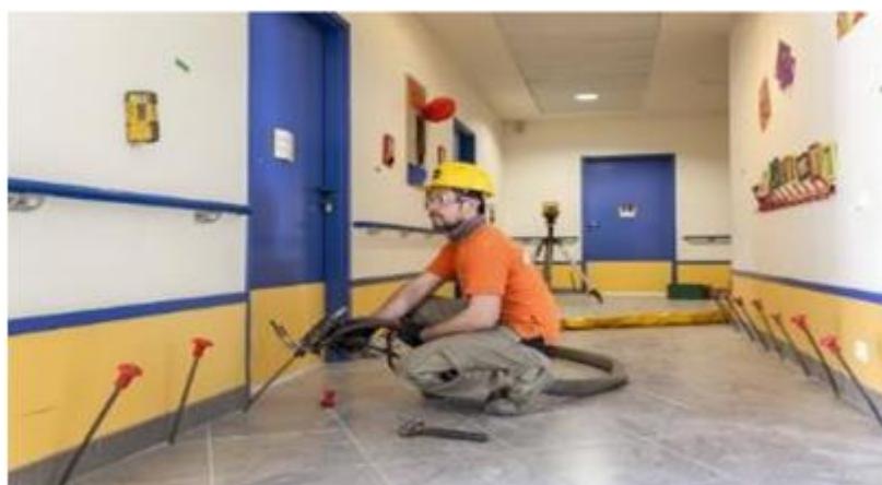
Figure 10: Expanding resin injection technique in the foundation soil.
