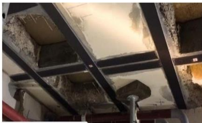
Figure 21: Floor reinforcement with CFRP composite material
