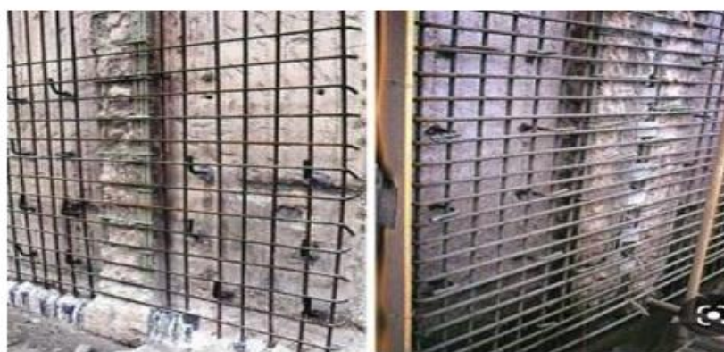
Figure 17: lining of reinforced concrete walls.
