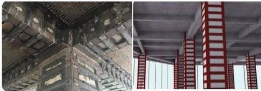
Figure 13: cracks protections
