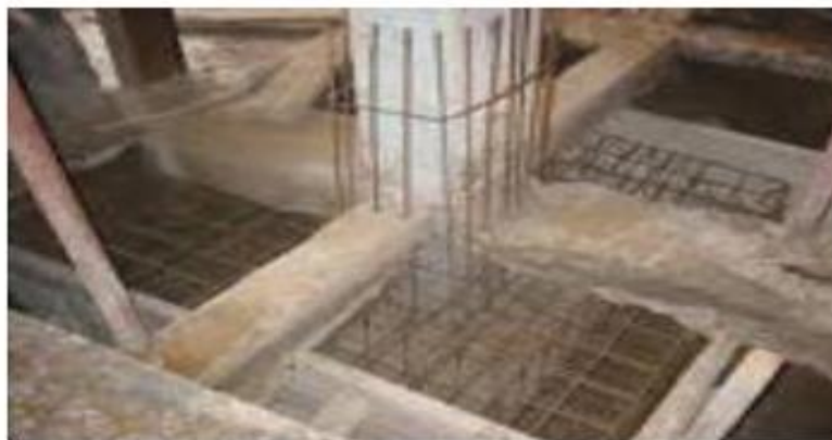
Figure 10: micro piles reinforcement of foundations.
